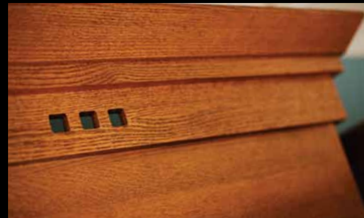
The molding stack uses a beveled crown with the carved "3-square" motif.
