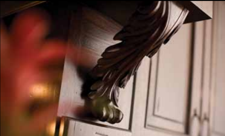
A corbel shaped like a palm frond was selected for the mantel hood.
