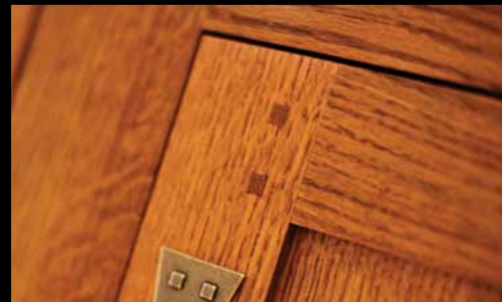
Originally a joinery technique, square pegs are now used as a decorative element.
